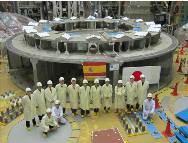
Figure 2: In front of the cryostat base
