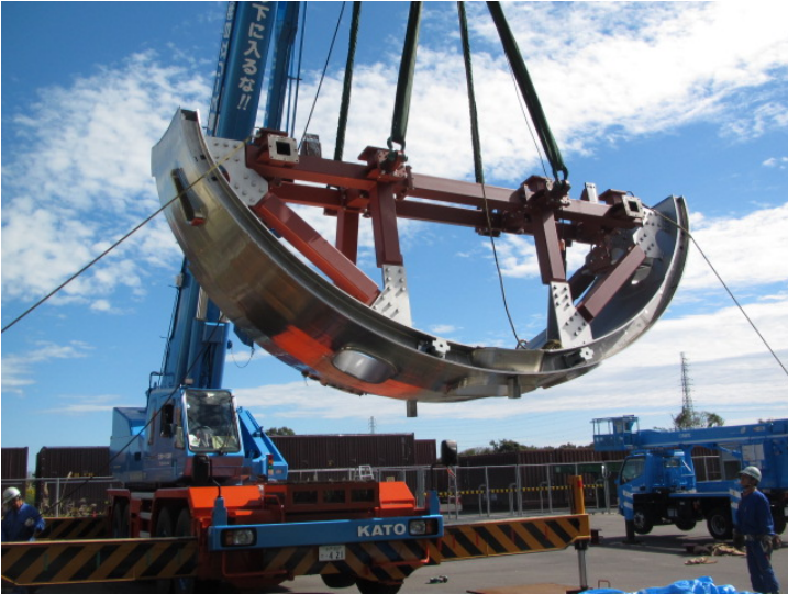
Figure 1: The eighth 30° outer sector unloading from the truck
